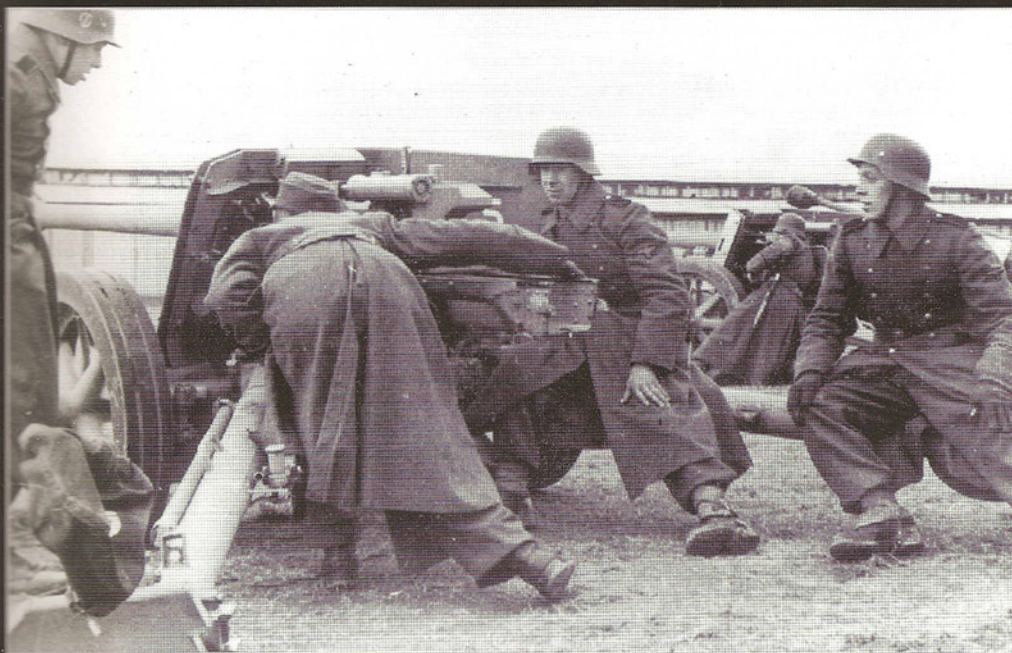
[Left] Training the SS gun crews. PaK 40's low profile has its disadvantages, aiming the gun is an awkward job. The wheels on the two guns have different spokes. The muzzle cover is draped over the folding handle on the spade. Like the one on the gun in the background, it has a number in white, corresponding with the number on the inside of the gun shield. These muzzle covers are simple bags, without the stiff front seen in an earlier photograph. Both gunners are pulling or pushing the gun, this may be a way to speed traverse and thus aiming the gun. The man on the right and the gunner of the gun in the back have cuff titles on their greatcoats. Take notice of the different style of gaiter worn by the man on the right. [Zbigniew Lalak Collection]
